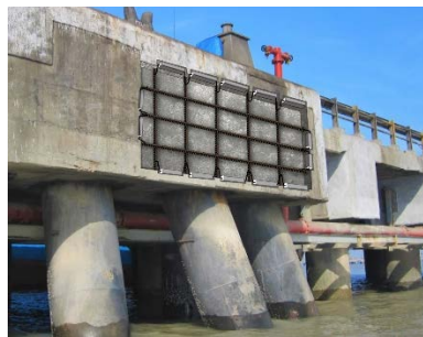
SMART ZINC® 130 Edge anodes installed in the parent concrete along the perimeter of the repair patch.
