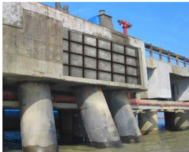
Exposed and cleaned steel reinforcement.
