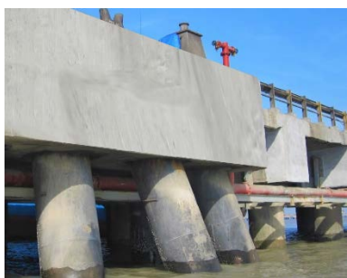
Repaired concrete structure.
