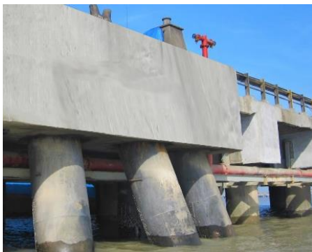
Anode encapsulated with repair mortar.
